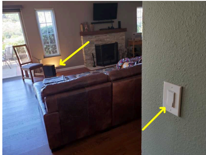
Dimmer switch and associated receptacle
