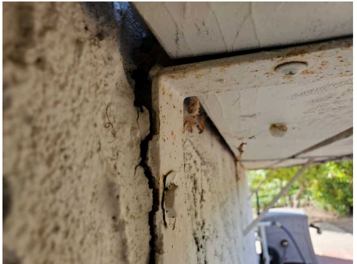
Gap at stucco and shelf brace
