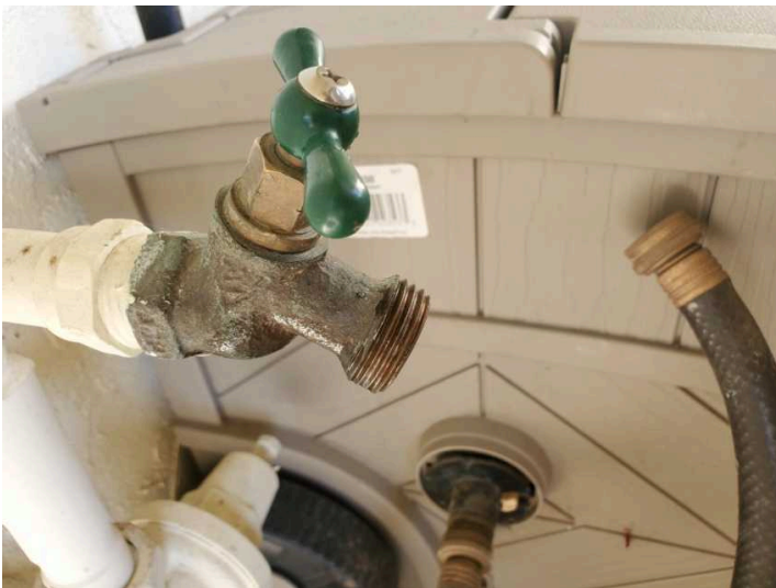
Missing anti-siphon valve
