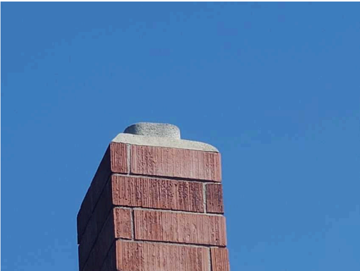
No rain cap/spark arrestor
