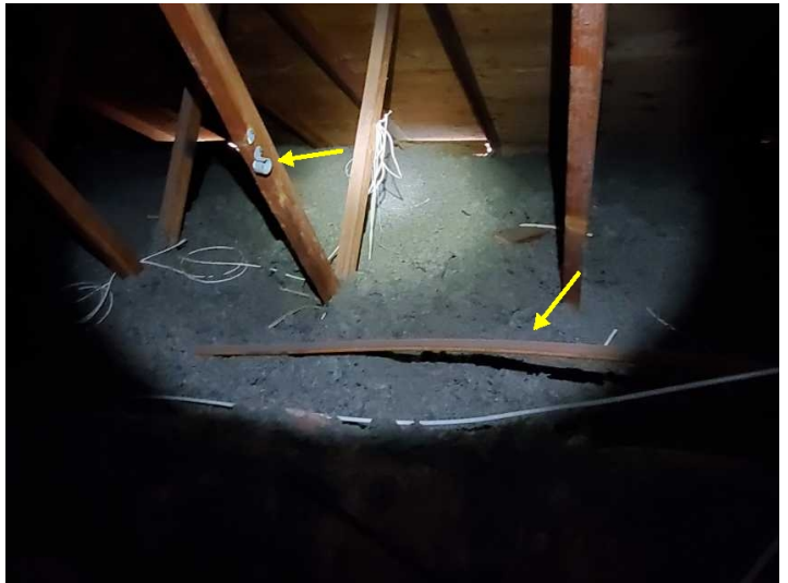
Broken support and unsecured piping
