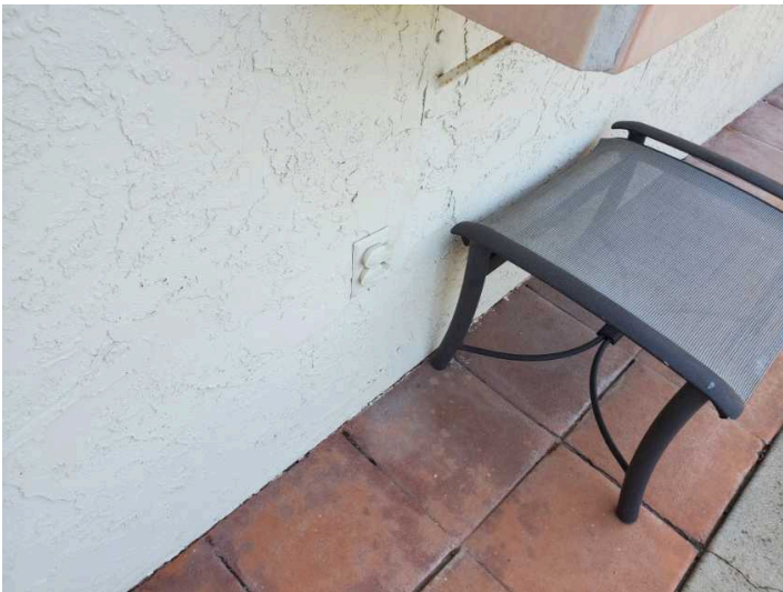
In-use cover not installed
