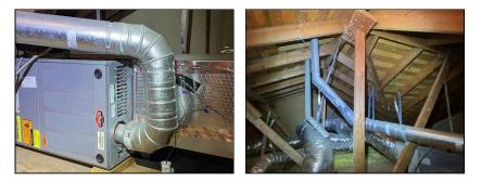
7.4 Cooling and Air Handler Equipment Comments: Acceptable CONDENSER UNIT MANUFACTURER - HEIL MANUFACTUR DATE - 07/2016 TON CAPACITY - 3 TON MODEL # NH4A436AKA100 SERIAL # X163088302 HFC - 410A
