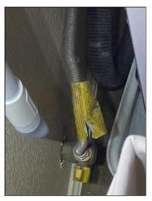
5.2 Dryer vented & vent type Comments: Acceptable Flexible steel dryer vent pipe
